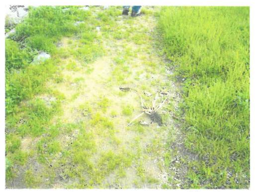
Photograph 19 - Sparse vegetation along upstream slope of left embankment
