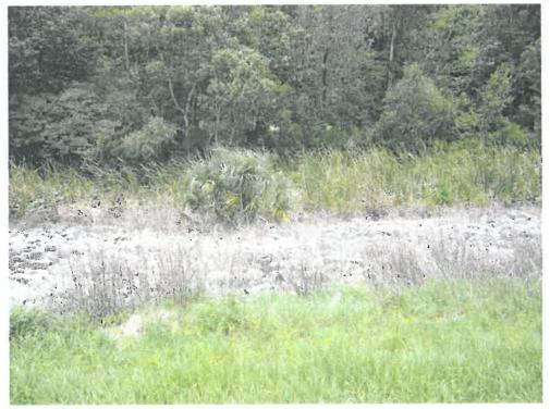
Photograph 26 - Palm tree located on the downstream slope of the right embankment
