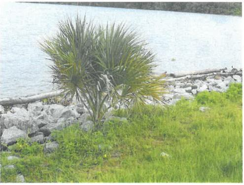
Photograph 20 – Palm tree on upstream slope that should be removed
