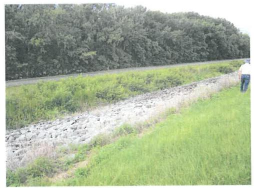
Photograph 21 – Heavy vegetation along the rip rap revetment of the left embankment
